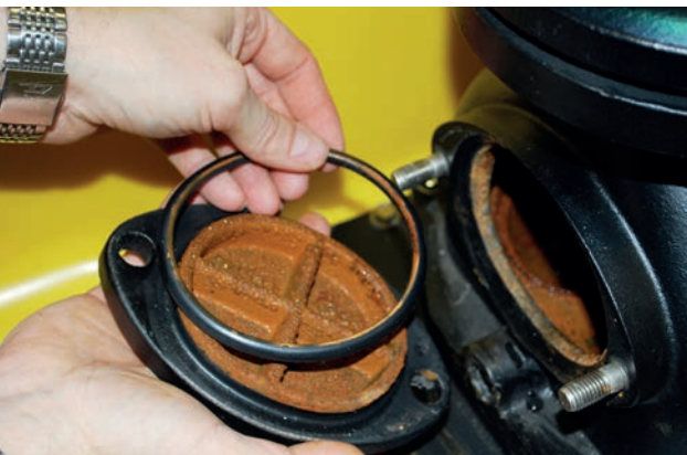
▶ Checking and cleaning the swing-type check valve
